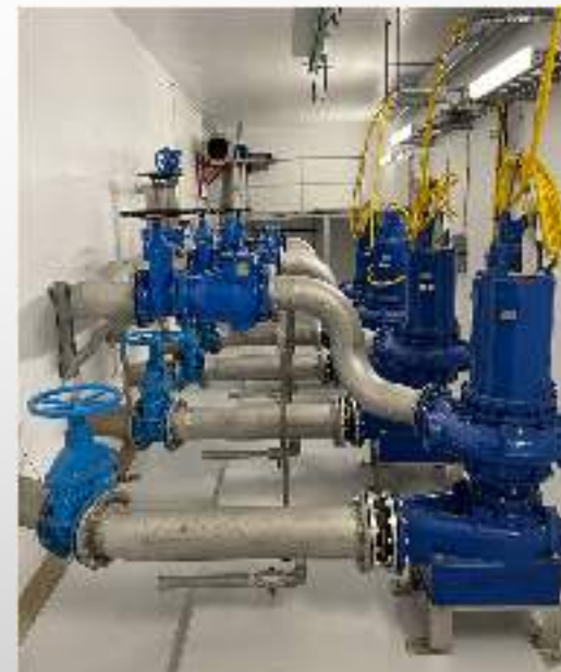
Ferdig rehabilitert i 2022
