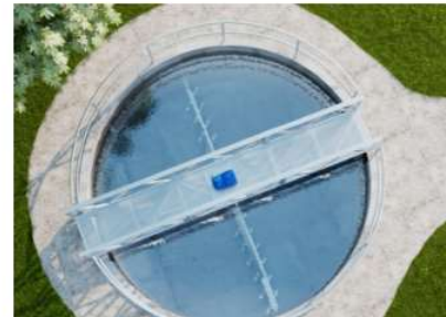
Picket Fence Thickener (Gravity Thickener)
