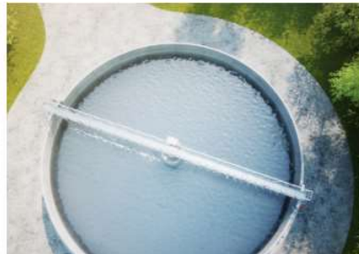
Rotating sludge scraper
