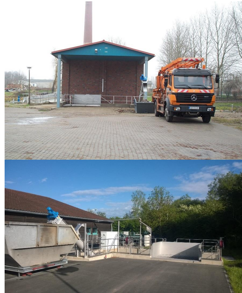
Grit acceptance tank on different WWTPs
